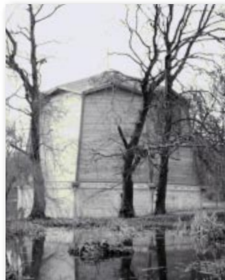
The Djamichunatra, a nine-sided building designed according to Gurdjieff principles. Later used for Subud latihans and Bapak talks.
