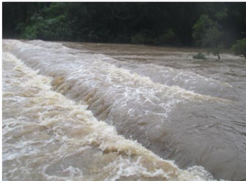
Bridge across the Tweed River.
