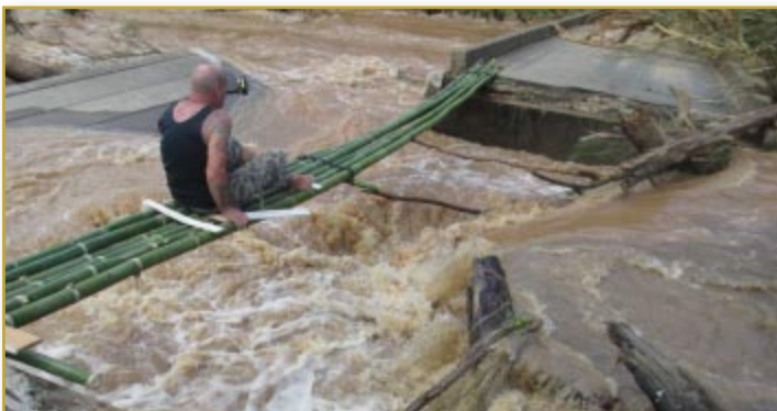
A volunteer constructs a bamboo link over the missing section of the bridge across the Tweed River. The idea is we might be able to walk out on it, but today rain is falling again, and conditions are unpredictable.
