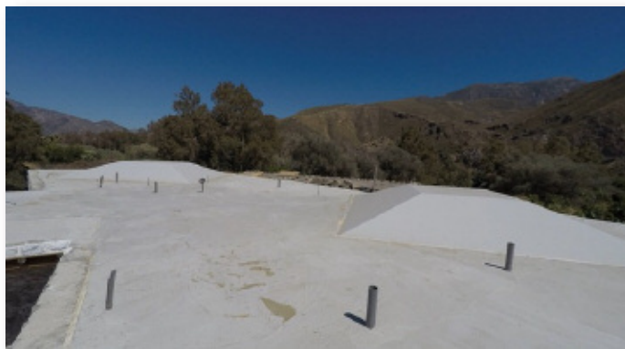
Latihan Hall under construction in Orgiva.
