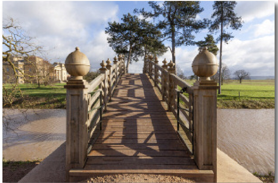
Included amongst Green Oak's many public projects are a number of traditional oak bridges.
