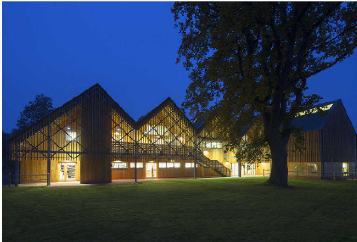
The Art and Design block of the Bedales School. Green Oak has carried out several educational projects.
