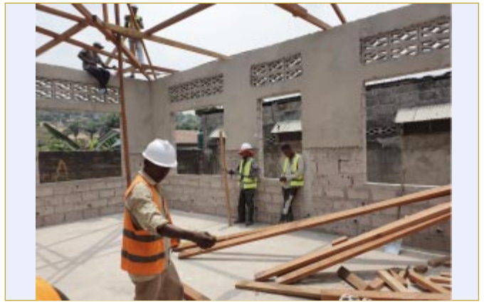
Kinshasa – Lemba Imbu - new pediatric clinic under construction.
