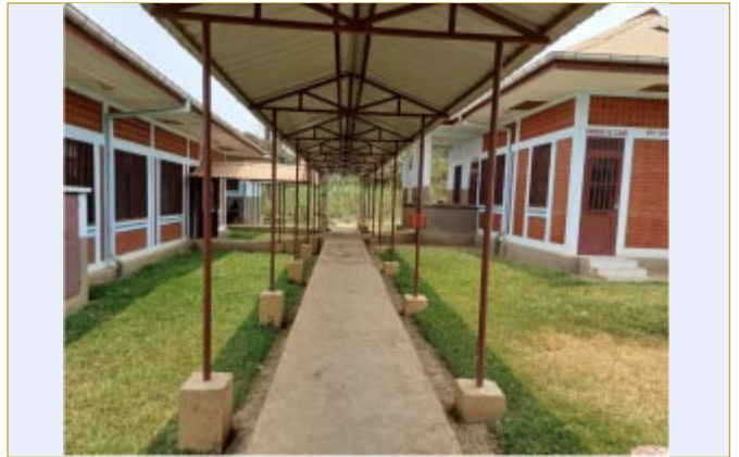
The KN Reference clinic with a canopy to the pediatric clinic, left, the Radiology, and the laboratory, right.
