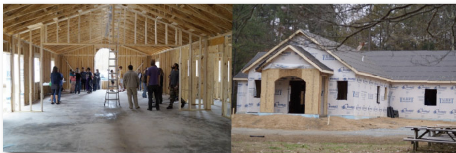
Blue Dove House under construction.
