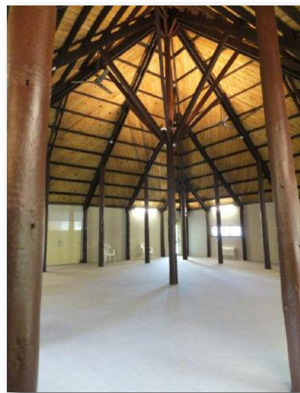
Work completed on the Grand Hall in Christchurch.
