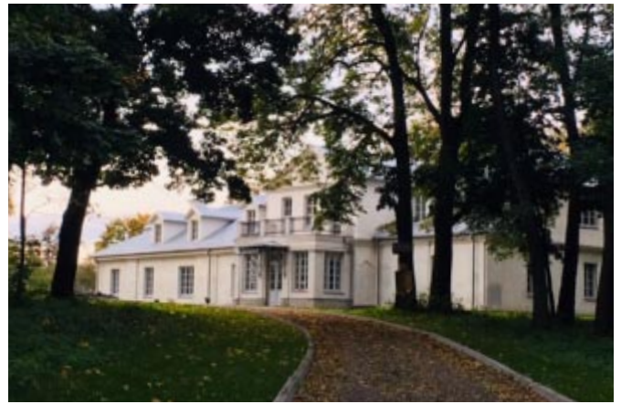
Approaching the main building.
