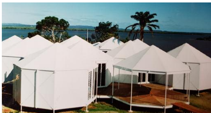
Ludwig Goetz based the design of his house on Bedouin tents he had seen in the deserts of Saudi Arabia.
