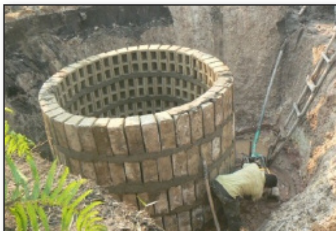
Well under construction.
