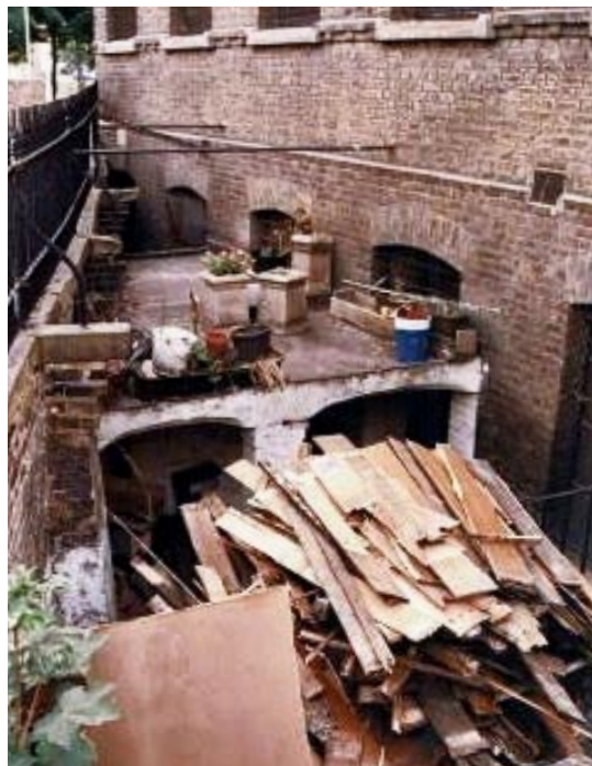
Clearing out in progress.
