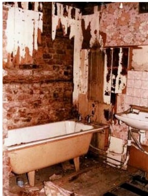
day washing dirty mugs. I found a Much to be renovated..
