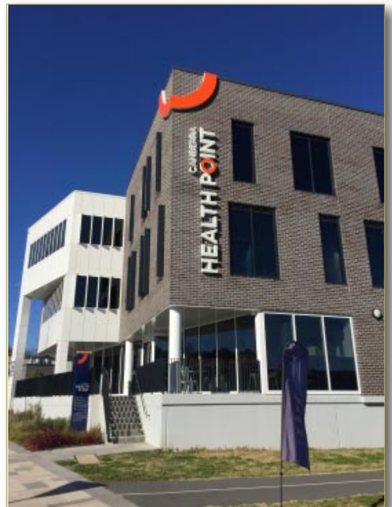
Canberra Health Point, which is a two-storey building, dedicated to health clinics. (By Harry Armytage.)
