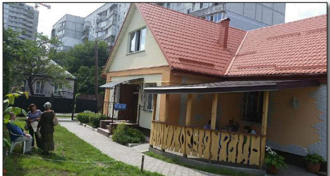
The Cherkassy Subud House. How it looks now, after the installation of heat insulation of its walls and other external jobs, which we were able to afford solely thanks to grants from MSF. (Photo by Viktor Boehm)
