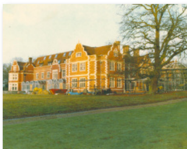
Anugraha under construction.
